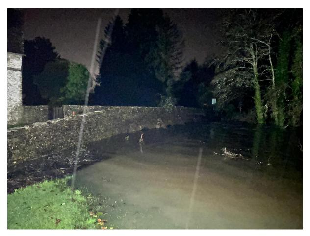
In effect the bridge, once the water rises sufficiently, acts as a dam causing the water to back up into the centre of the village causing a potential serious flood issue to residential properties. To date this has not occurred but any increase in surface water entering the river upstream from Easton Grey increases that risk.
